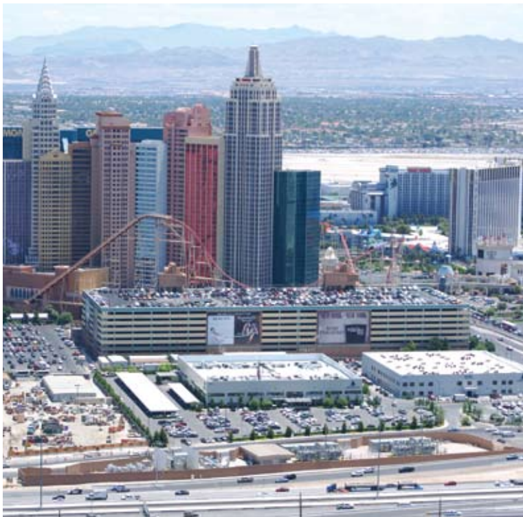
Aerial view of the Sinatra substation looking toward the strip.
