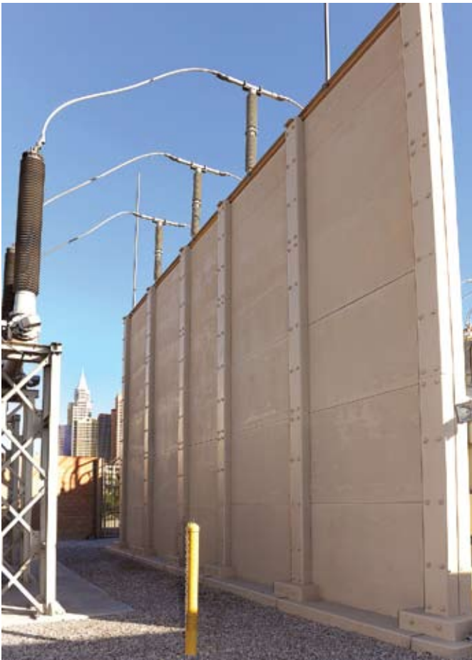
The firewall is restored and none the worse for having lived up to its design function.
